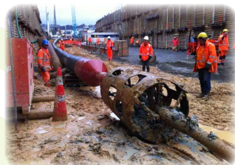
▲ The 710mm diameter polyethylene pipe is connected to the barrel reamer and drill string ready for installation
