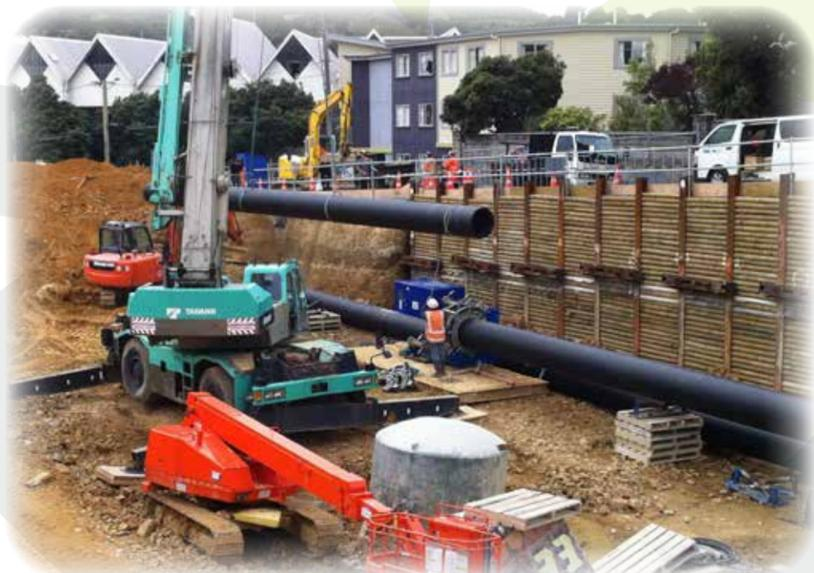
In tandem with the tunnel opening operation the 710mm diameter, SDR 11 polyethylene pipe was delivered and welded into two 100m long pipe strings. Once welded and tested they were positioned ready to be pulled into the tunnel. The front end of one string was fitted with a steel towing cone and connected to the drill string.
