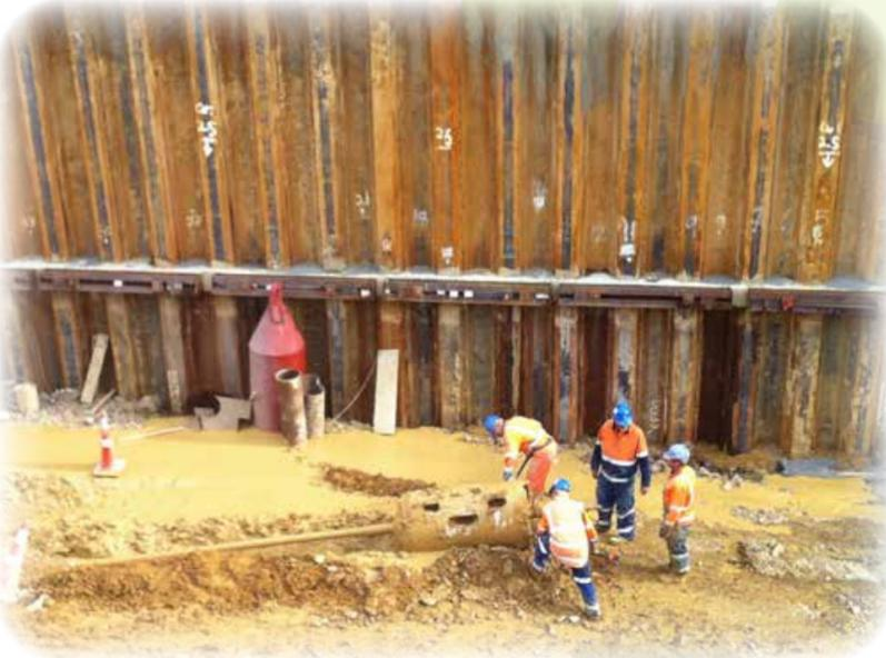
▲ Barrel reamer utilised to counter sinkage in the soft ground sections of the 200m long drill shot
