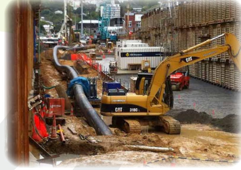
On completion of the pipe installation a cement plug was pumped around the pipe at each end to control ground water tracking along the outside of the pipe. The pipeline was pressure tested, CCTV undertaken and handed over to the alliance.
