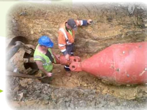
▶ Connecting the towing head to the swivel
